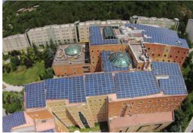
Solar energy system on the roofs of buildings in Yeditepe University campus with the capacity of 1 MW using 3850 Axitec solar panels with Huawei inverters
